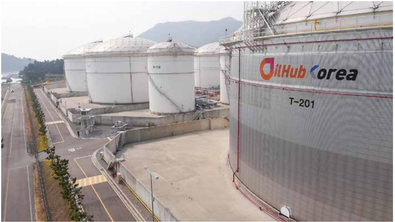
OKYC storage facilities OKYC的储罐设施
