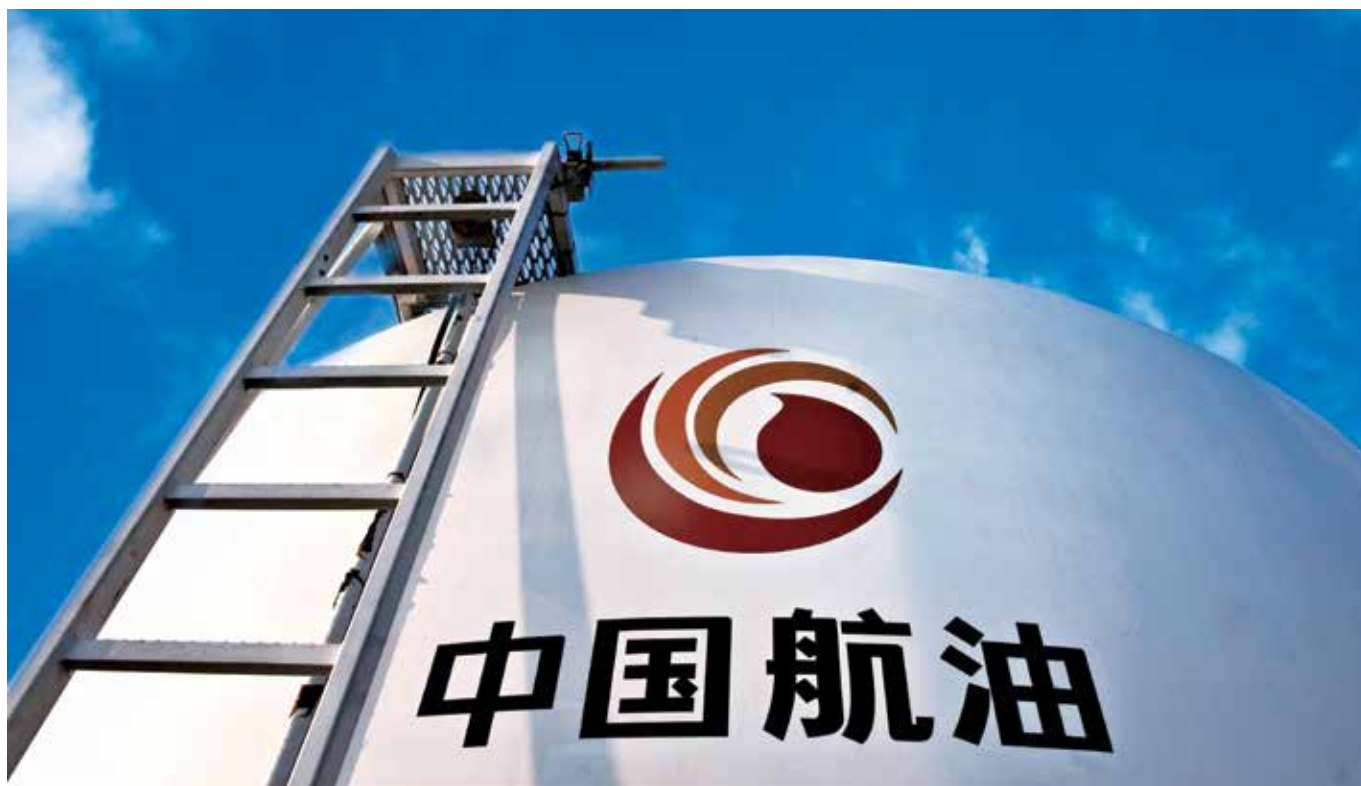
Oil storage facilities at CNAF CNAF储罐设施
