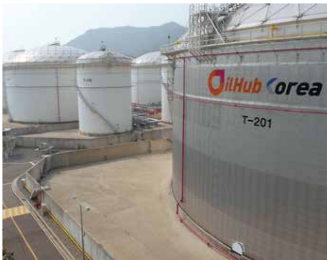
OKYC storage facilities OKYC的储罐设施
