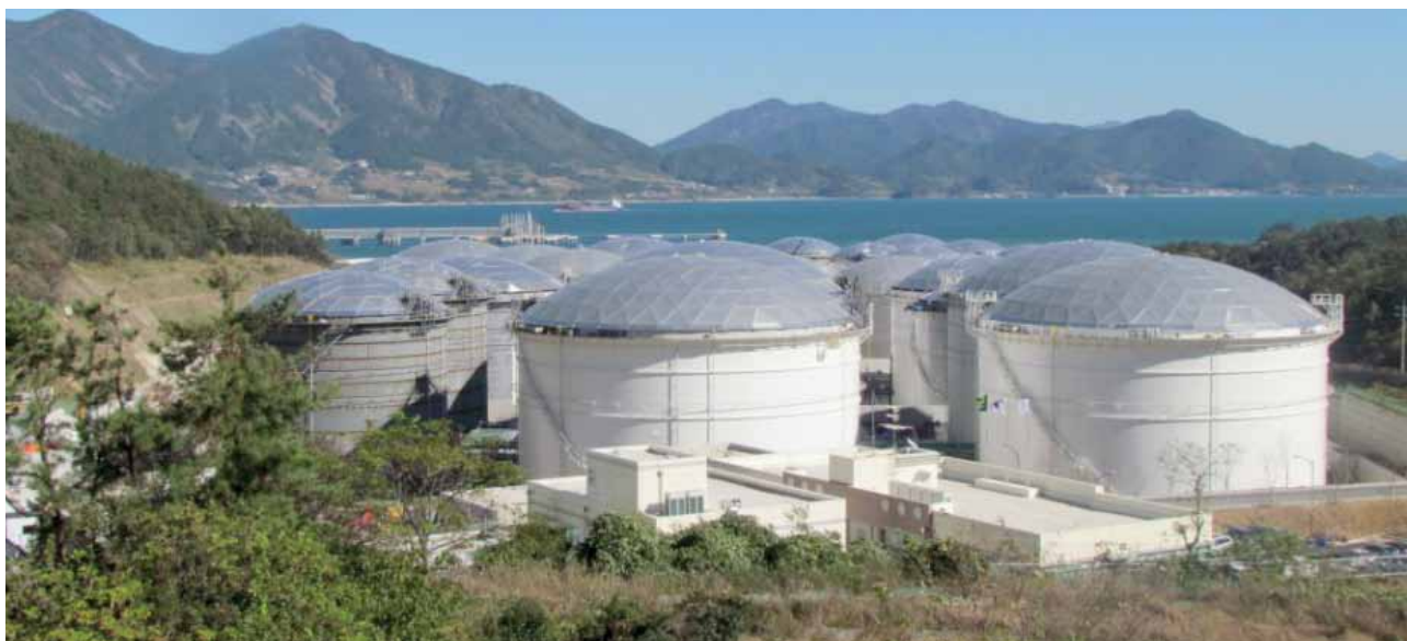
Storage facilities at OKYC OKYC储罐
