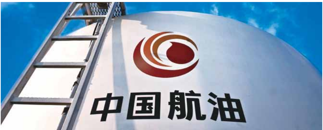
Oil storage facilities at CNAF CNAF 储罐设施
